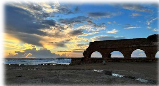
Herodian Aqueduct at Caesarea Maritima
